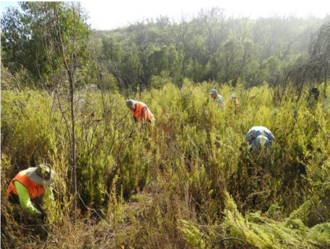
Below left: The team knocking out Erica below their lignotubers along Viminaria Creek.
